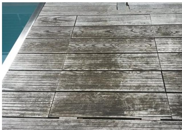
Figure 1: Thermally modified ash with discolouration by blue stain and mould
