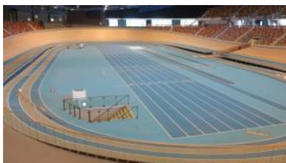
Figure 1: Cycle track with on the right an opening where the shutter is removed.
