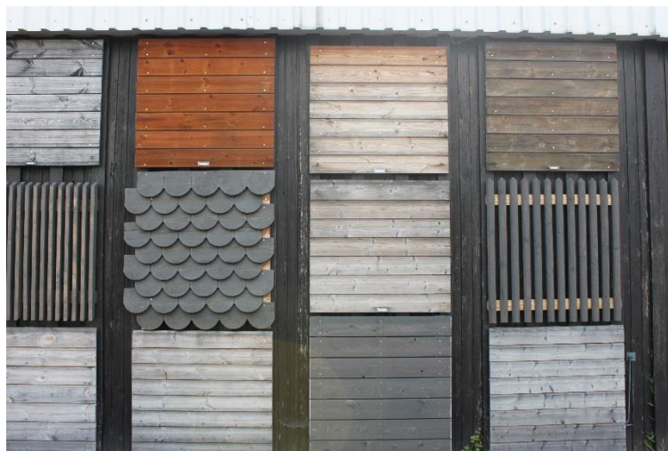
Figure 1: Exterior cladding test set up at Georg-August-Universität Göttingen in Germany.
