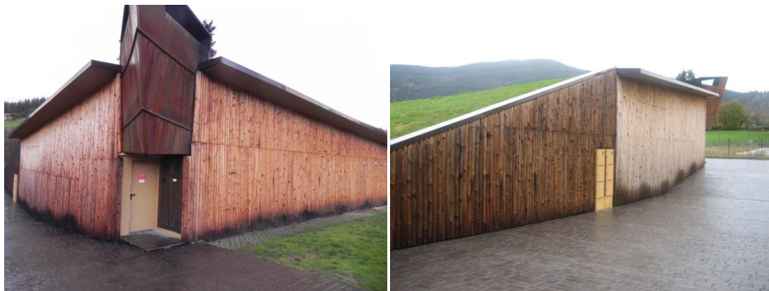
Figures 6 and 7: Different views of the thermal modified round radiata pine in Orozko.
