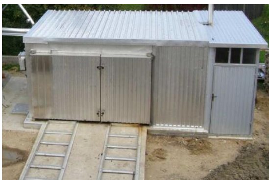
Figure 1: Chamber for thermal modification of wood, Hamech (model PW-10)
