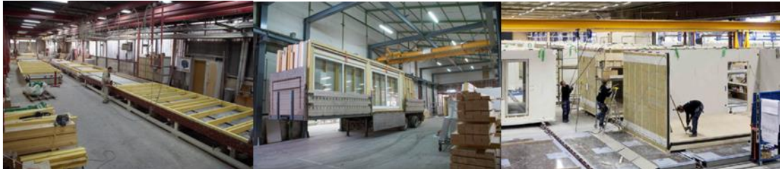
Figure 2: Examples of off-site prefabrication. Left to right: Manufacture of wall elements; Window sections ready for transportation to the building site; Manufacture of modules for a modular system.
