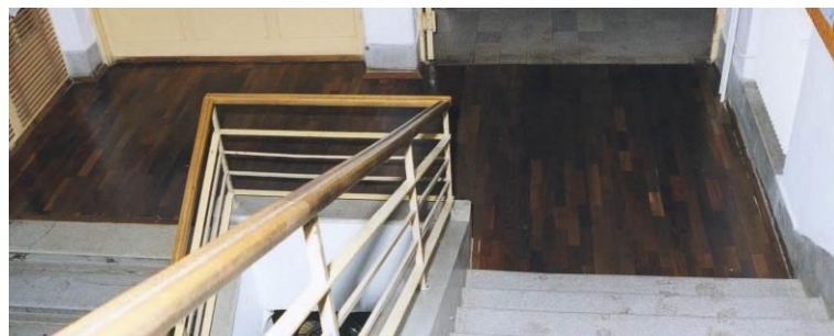
Figure 1: The appearance of the floor after installation
